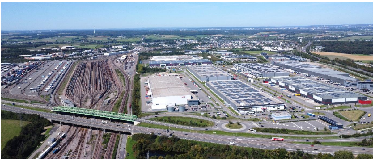
The Eurohub Sud in Dudelange harbours 150.000 sqm of warehouse space in a state-of-the-art multimodal platform (© Malik Zeniti/C4L)
